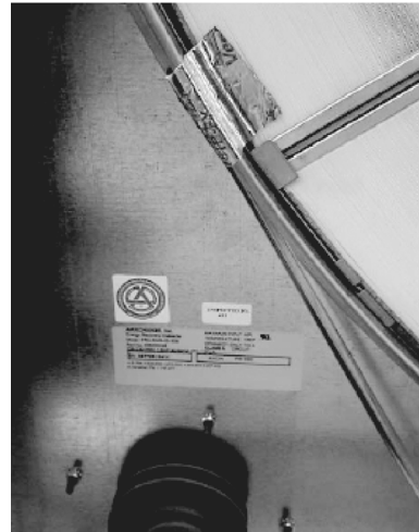
Figure 104. Link belt installation
