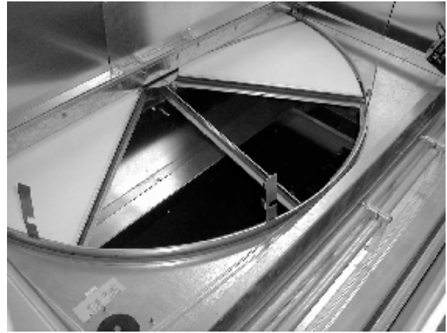
Figure 101. Segment Removal
