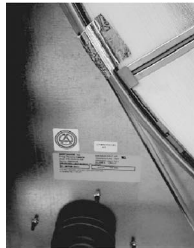
Figure 104. Link belt installation
