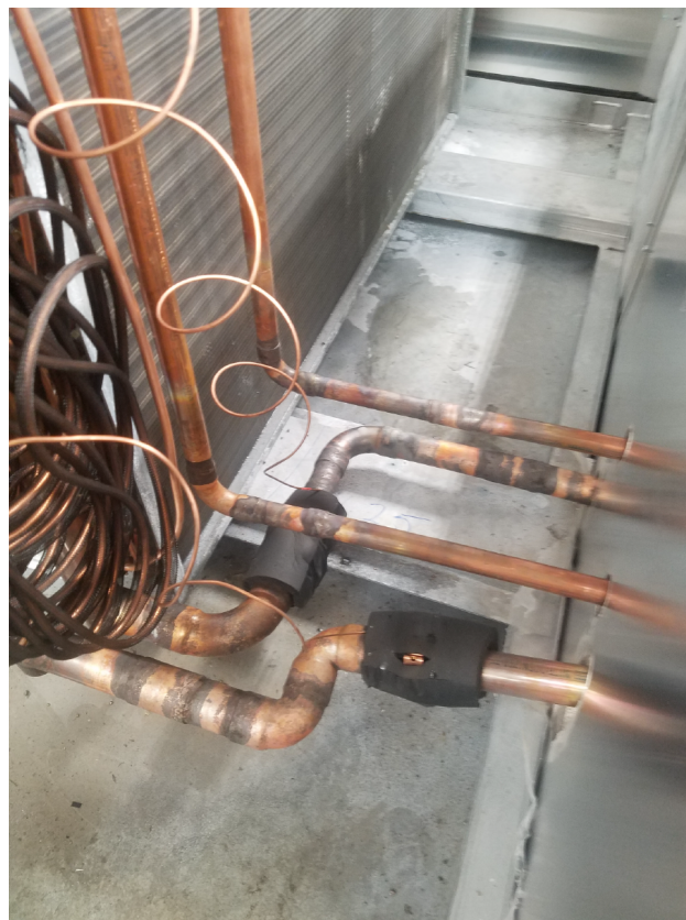
Figure 26. Braze suction and liquid lines
