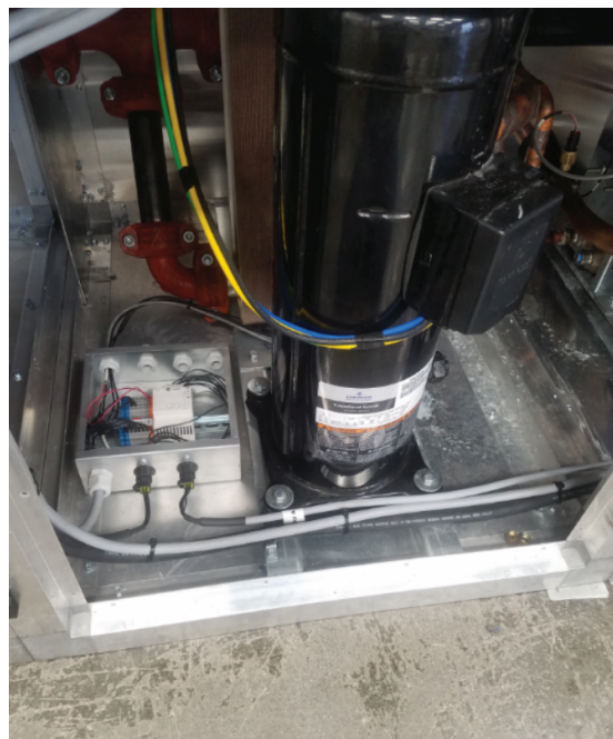
Figure 28. Variable speed power and communication wiring
