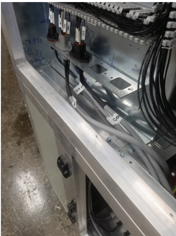
Figure 30. Compressor communication terminations
