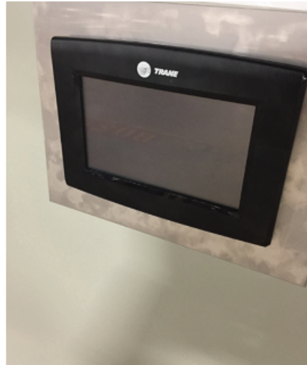
Figure 42. TD-7 Installation on front
