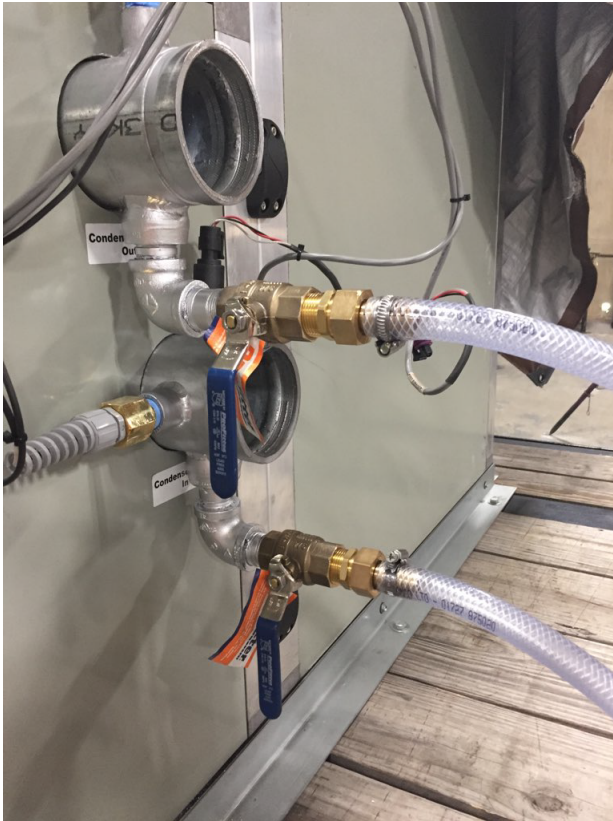
Figure 58. Typical setup for clean in place
