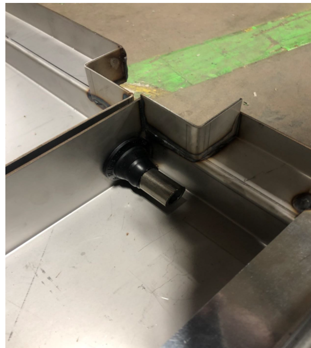
Figure 23. Joined drain pan installation
