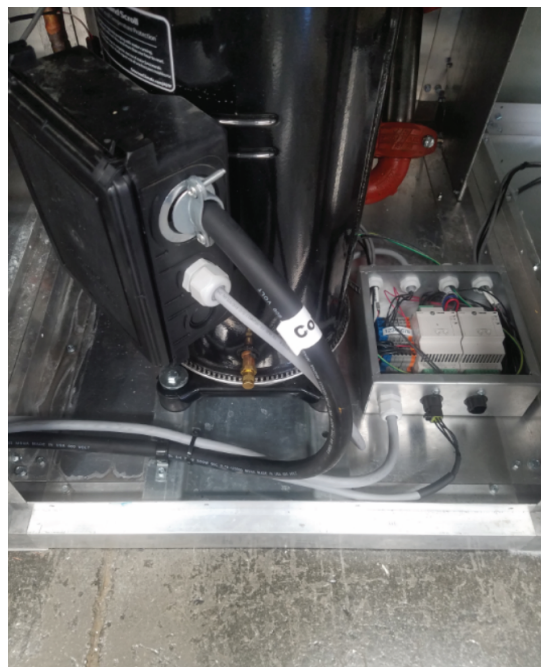
Figure 28. Variable speed power and communication wiring
