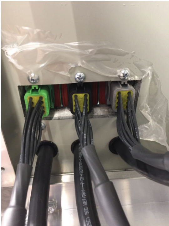
Figure 37. Fan power terminations
