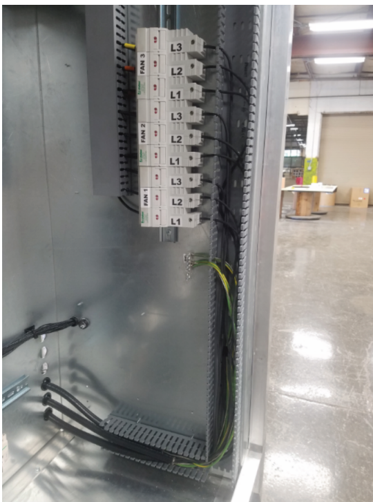
Figure 37. Fan power terminations
