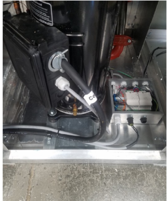
Figure 28. Variable speed power and communication wiring
