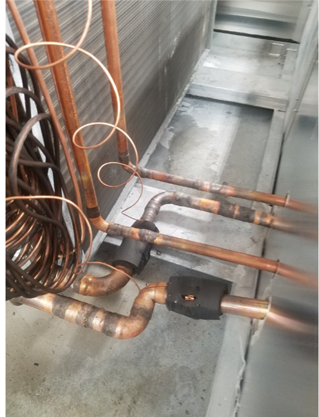
Figure 26. Braze suction and liquid lines
