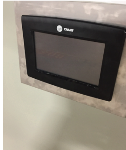
Figure 42. TD-7 Installation on front
