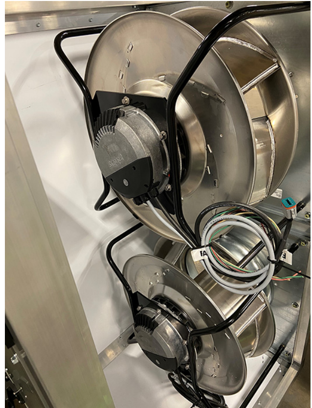
Figure 34. Fan power and communication wire routing
