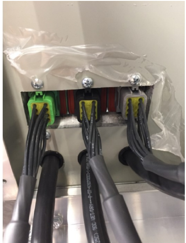
Figure 36. Fan communication terminations - pluggable connectors are color coded for ease of installation
