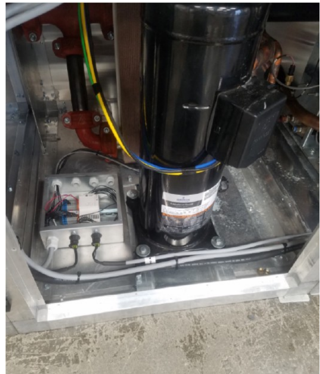
Figure 28. Variable speed power and communication wiring
