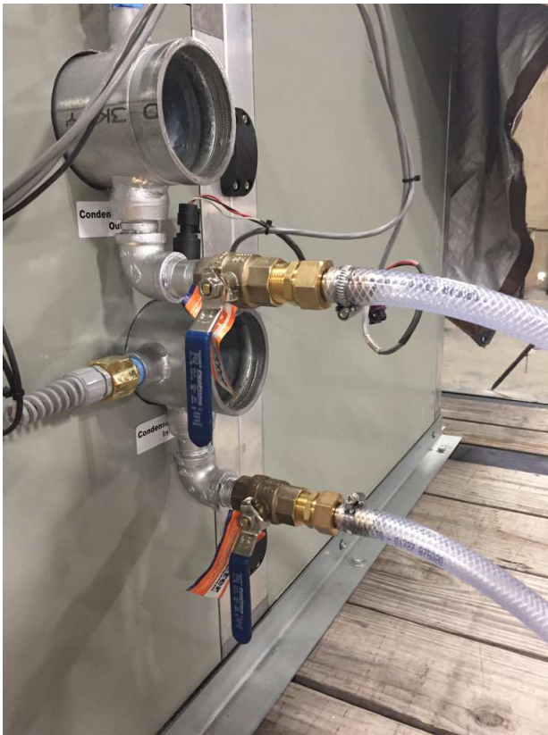
Figure 56. Typical setup for clean in place
