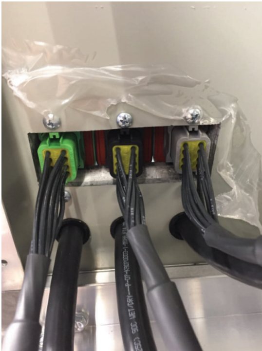
Figure 35. Fan power terminations
