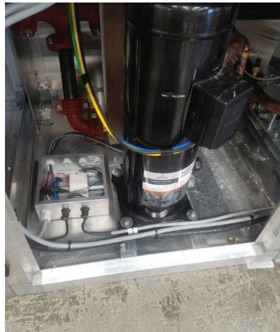
Figure 26. Variable speed power and communication wiring
