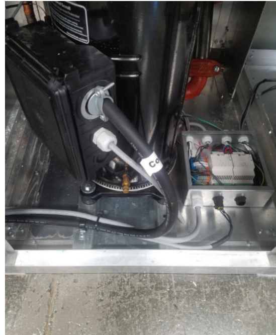
Figure 26. Variable speed power and communication wiring
