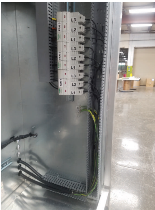
Figure 35. Fan power terminations
