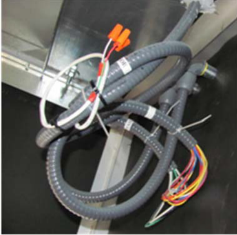
Figure 10. Reconnection extensions example
