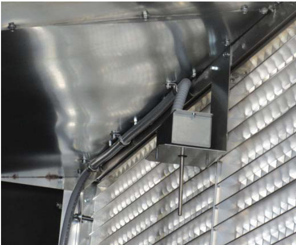
Figure 11. Typical control wiring - discharge temperature sensor (optional)
