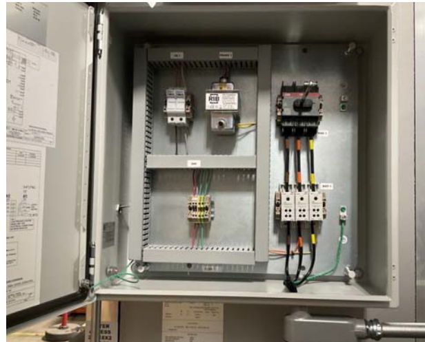
Figure 8. Typical power panel layout (options vary)
