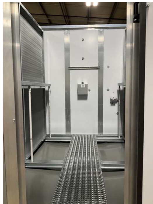
Figure 9. Unit interior (electrical reconnection)
