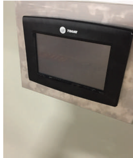
Figure 36. TD-7 Installation on front
