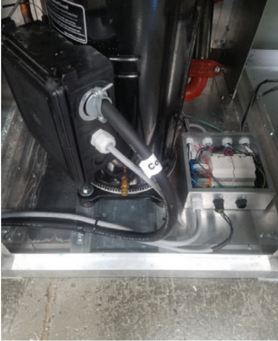
Figure 23. Variable speed power and communication wiring
