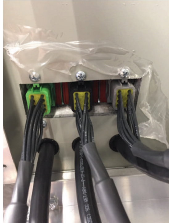
Figure 32. Fan power terminations
