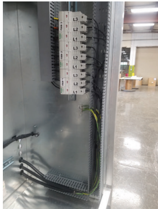
Figure 32. Fan power terminations
