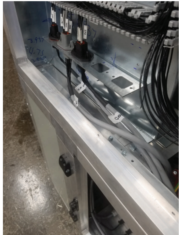
Figure 25. Compressor communication terminations
