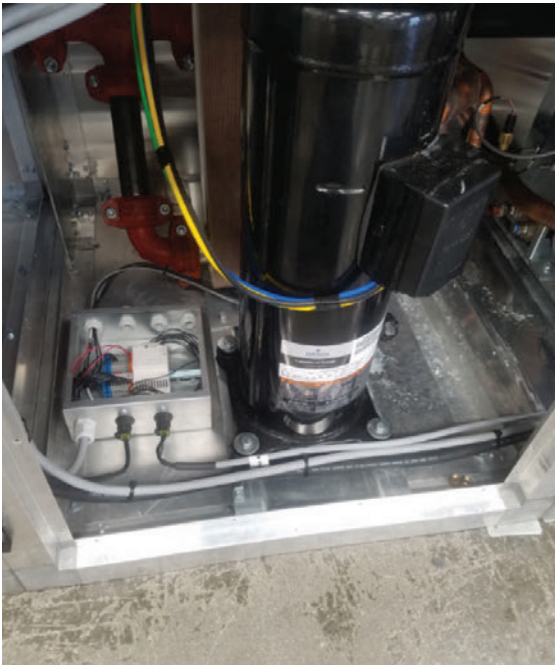
Figure 23. Variable speed power and communication wiring
