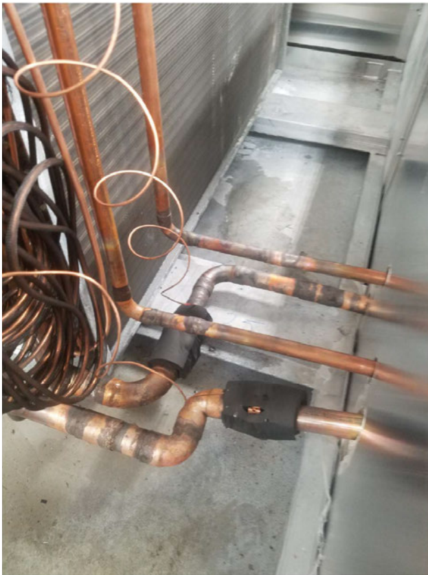
Figure 21. Braze suction and liquid lines
