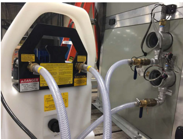
Figure 55. Rear view of Circulation pump
