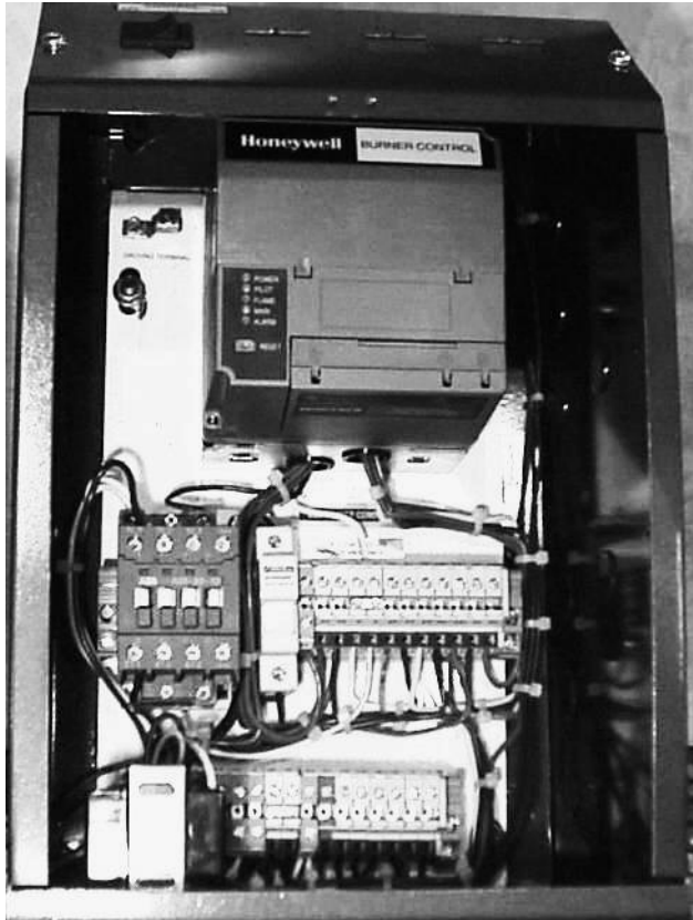
Figure 21. Control panel for the FDM burner on 1250 to 2400 MBh (20:1 turndown) units
