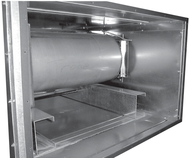
Figure 10. Entering airside (drum or primary) of gas heat section
