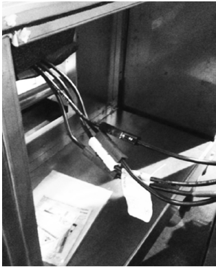
Figure 35. Horizontal section-to-section high voltage quick connects
