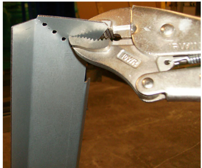
Figure 60. Bend end tabs, apply Butyl tape to flashing
