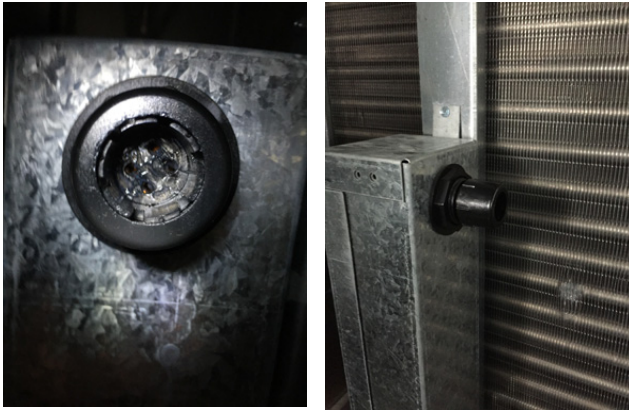
Figure 194. Plug pins into socket, then tighten compression nut
