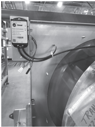
Figure 161. Typical transmitter install for DDP fans
