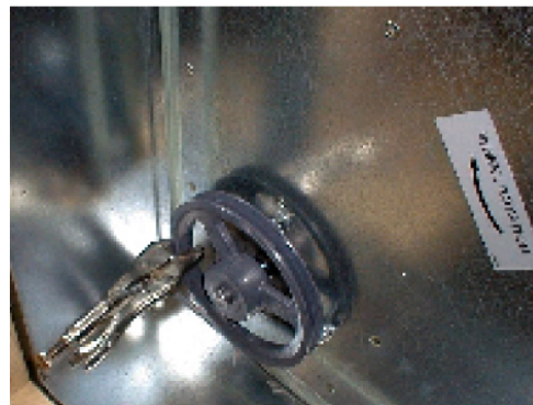
Figure 188. Secure pulley and belt with vise grip to prevent wheel rotation
