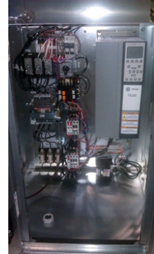
Figure 139. Internally mounted VFD
