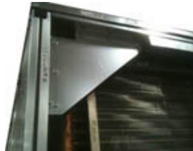
Figure 9. Shipping split seam – top view
