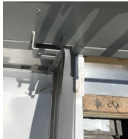
Figure 87. Pipe cabinet all thread at unit bracket detail
