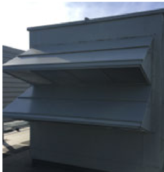
Figure 107. Front or back mounted multiple OA hood
