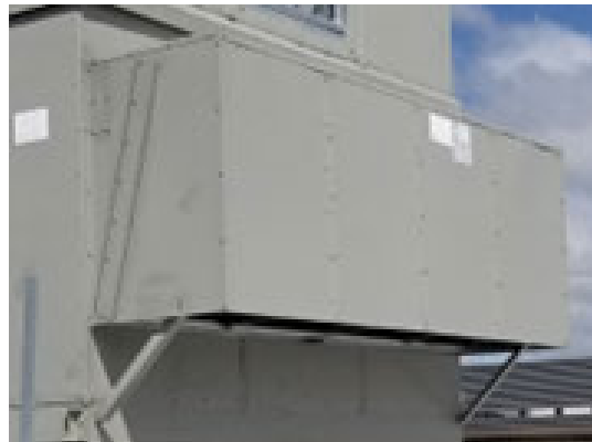
Figure 107. Front or back mounted multiple OA hood
