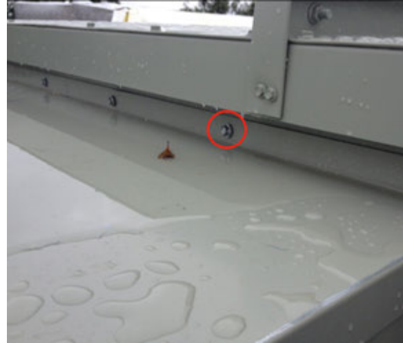
Figure 76. Pipe cabinet roof screw detail
