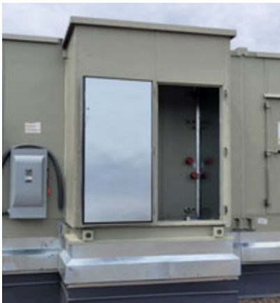
Figure 78. Pipe cabinet wide roof install
