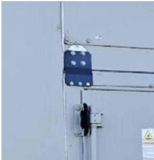
Figure 39. Stacking bracket installed
