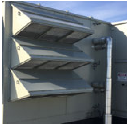
Figure 105. Side mounted multiple hood
