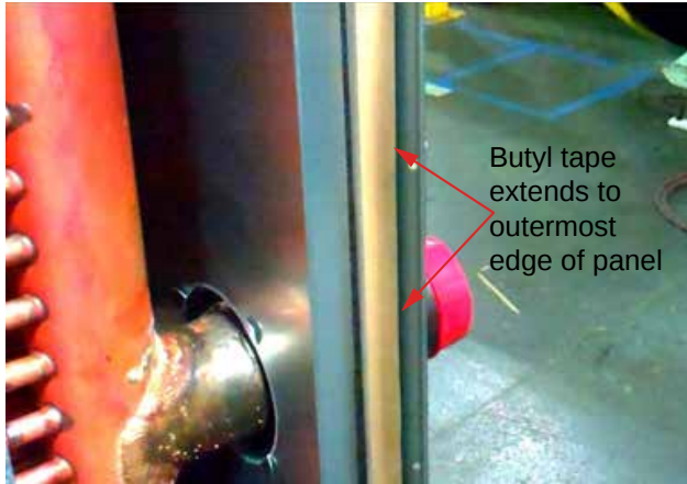
Figure 6. Install butyl tape on outdoor bases
