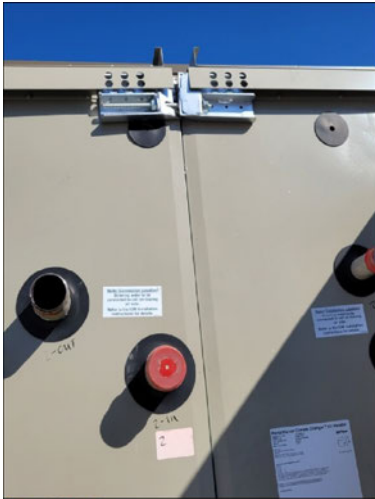
Figure 13. Right hand wedge block assembly – old design
