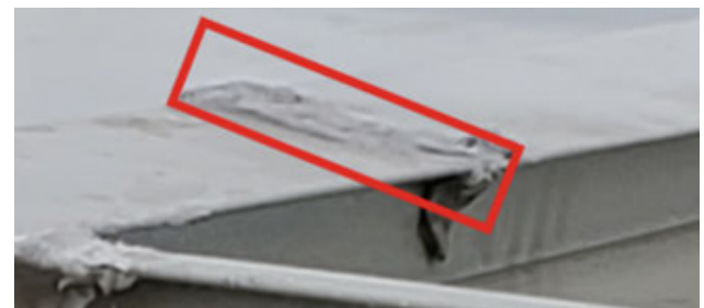
Figure 24. Two-piece wide roof strip caulk
