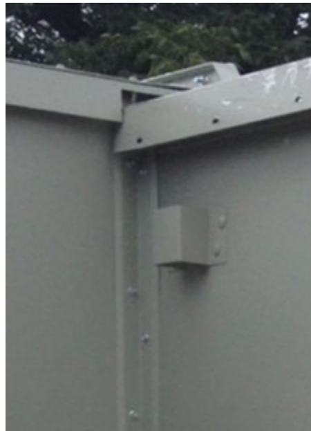
Figure 91. Pipe cabinet corner cap install
