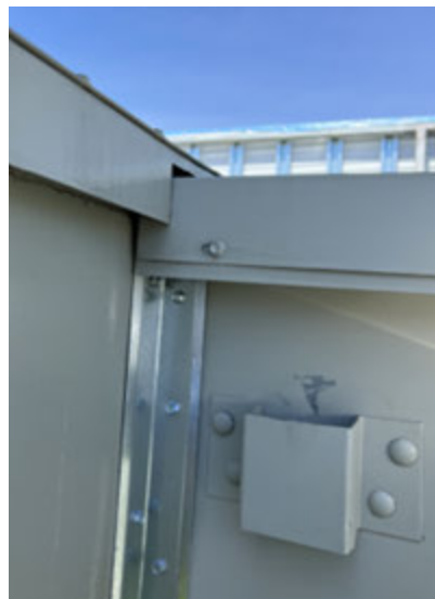
Figure 91. Pipe cabinet corner cap install
