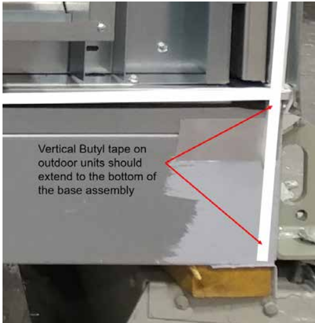
Figure 6. Install butyl tape on outdoor bases
