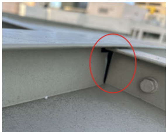
Figure 29. Vertical seam close-up
