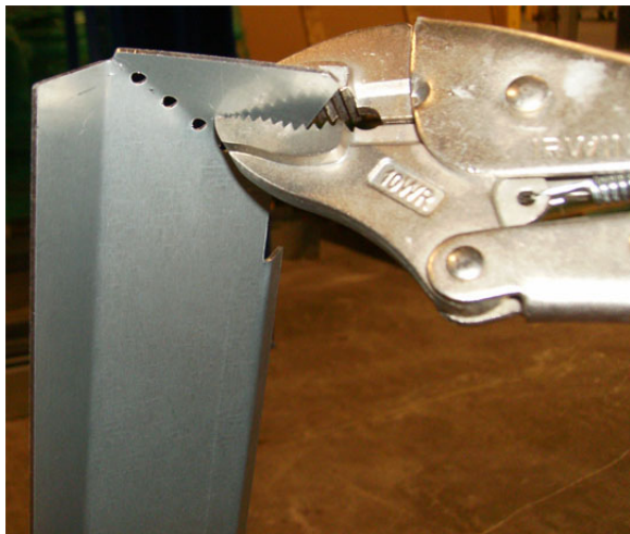
Figure 55. PTAF stacked flashing
