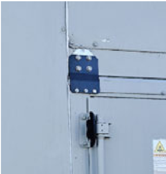
Figure 39. Stacking bracket installed
