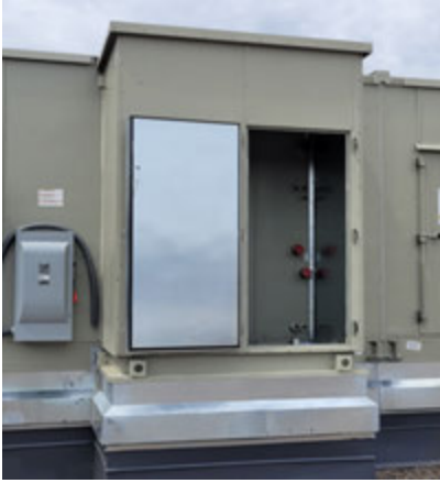
Figure 78. Pipe cabinet wide roof install
