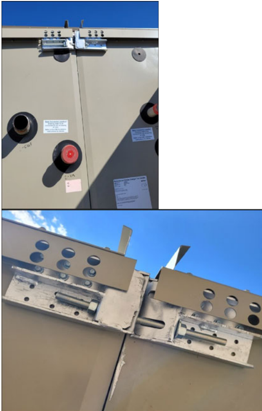
Figure 13. Right hand wedge block assembly – old design
