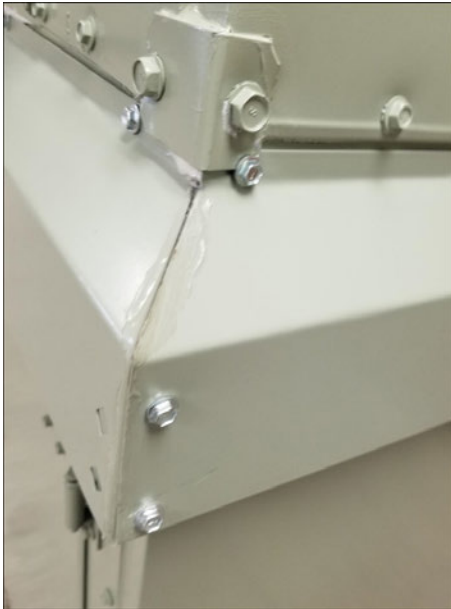
Figure 45. Stacked corner seam
