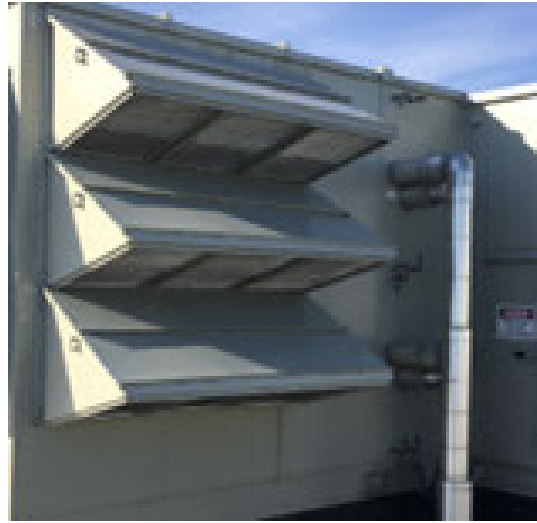
Figure 105. Side mounted multiple hood
