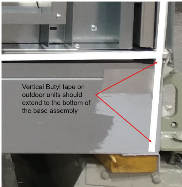
Figure 6. Install butyl tape on outdoor bases
