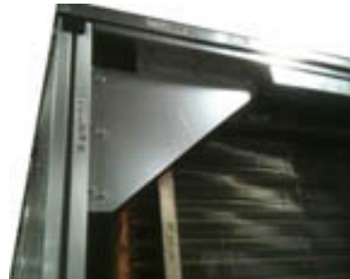
Figure 9. Shipping split seam – top view
