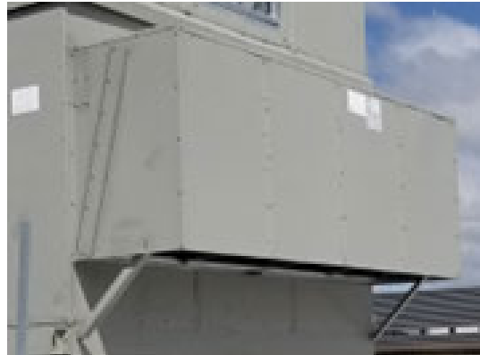
Figure 107. Front or back mounted multiple OA hood
