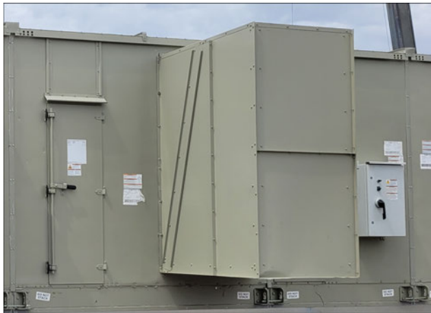
Figure 104. Side mounted OA hood
