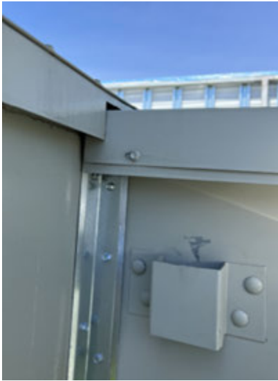
Figure 91. Pipe cabinet corner cap install
