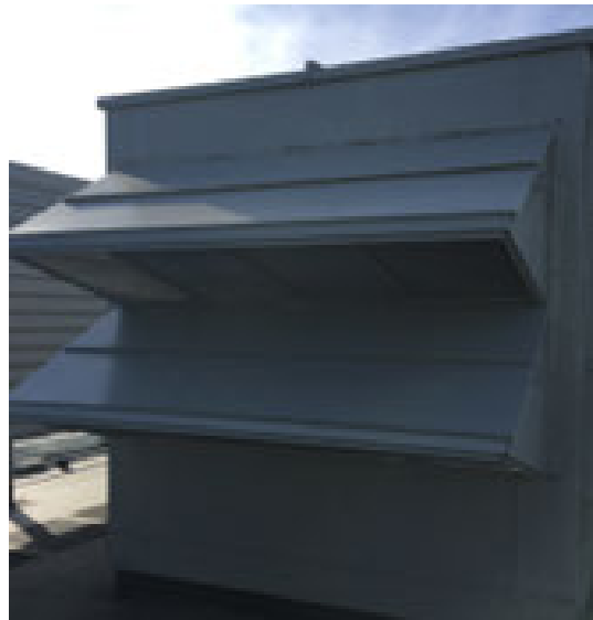
Figure 107. Front or back mounted multiple OA hood
