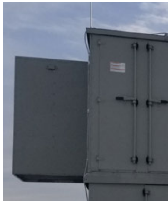
Fan Section side discharge exhaust hood installation (intake hood shape varies)
