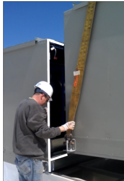
Figure 7. Shipping split lift
