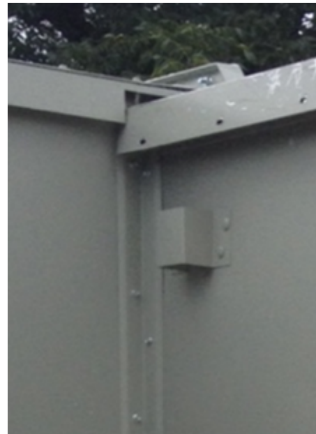
Figure 90. Pipe cabinet corner angle install
