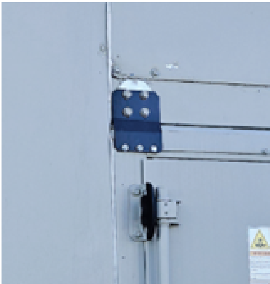
Figure 39. Stacking bracket installed
