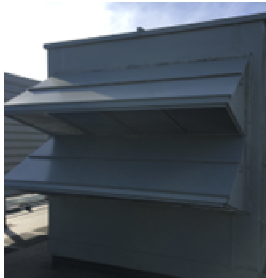
Figure 107. Front or back mounted multiple OA hood
