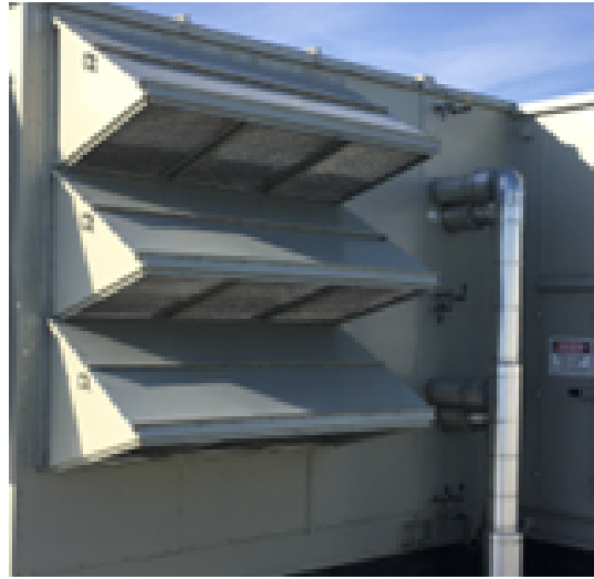
Figure 105. Side mounted multiple hood
