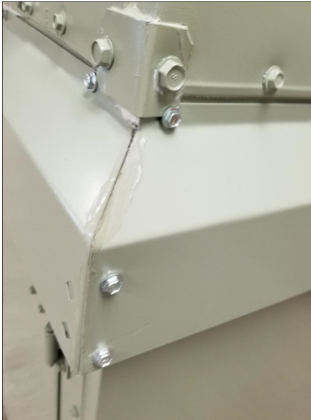
Figure 45. Stacked corner seam
