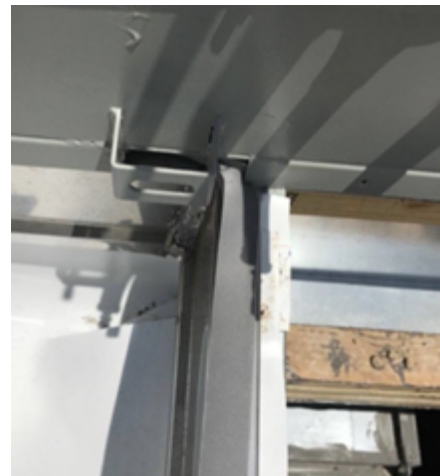
Figure 86. Pipe cabinet roof curb W bracket at unit base
