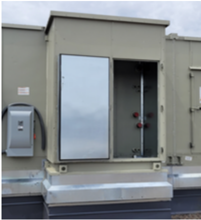
Figure 78. Pipe cabinet wide roof install
