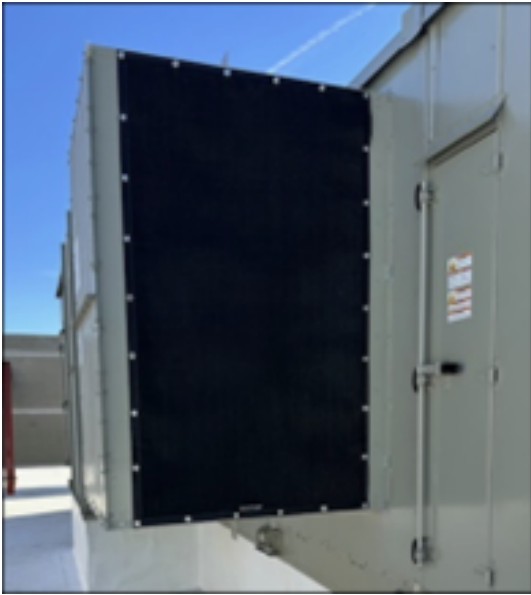
Figure 110. Fan section side discharge exhaust hood installation (intake hood shape varies)
