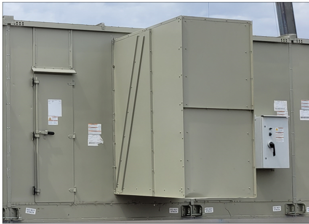
Figure 104. Side mounted OA hood
