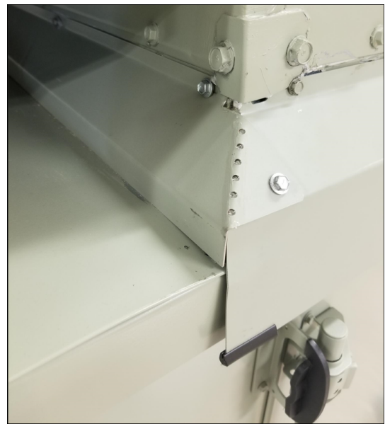
Figure 57. Caulk along seam
