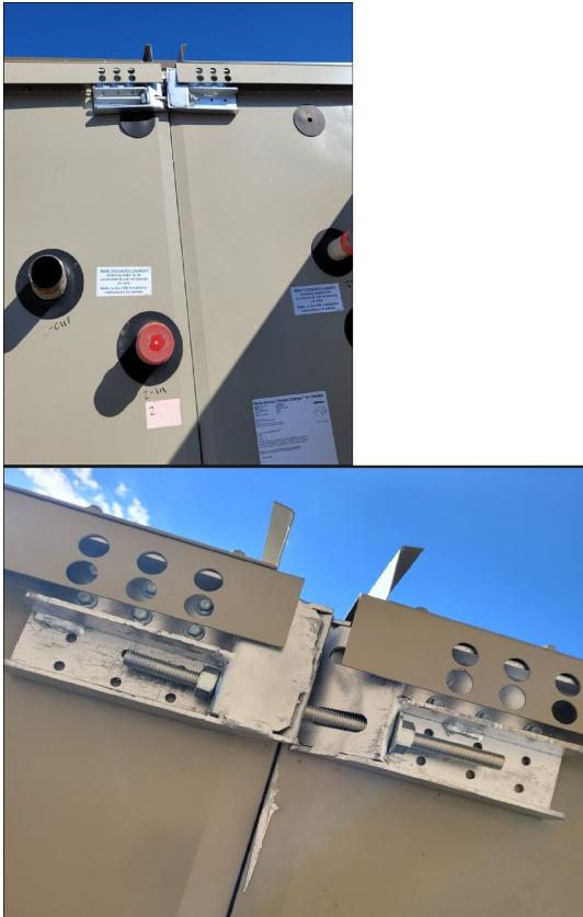
Figure 13. Right hand wedge block assembly – old design
