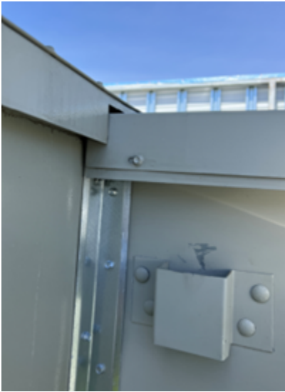
Figure 91. Pipe cabinet corner cap install
