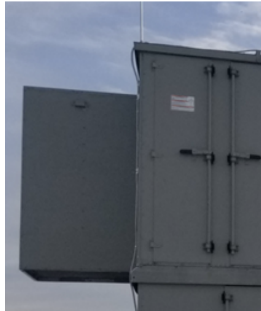
Fan Section side discharge exhaust hood installation (intake hood shape varies)
