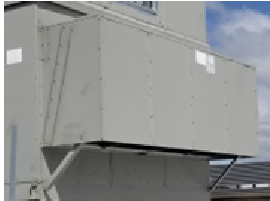
Figure 107. Front or back mounted multiple OA hood
