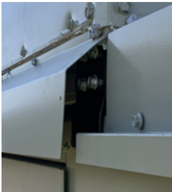
Figure 61. Stacked flashing to first level C-channel style roof
