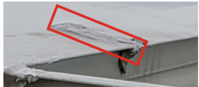
Figure 24. Two-piece wide roof strip caulk
