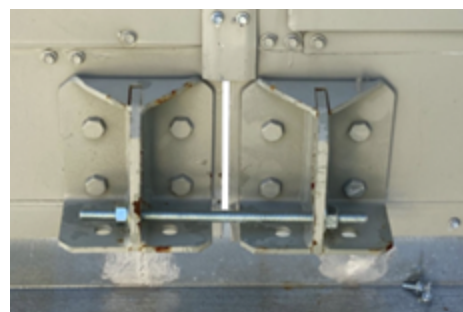
Figure 9. Shipping split seam – top view
