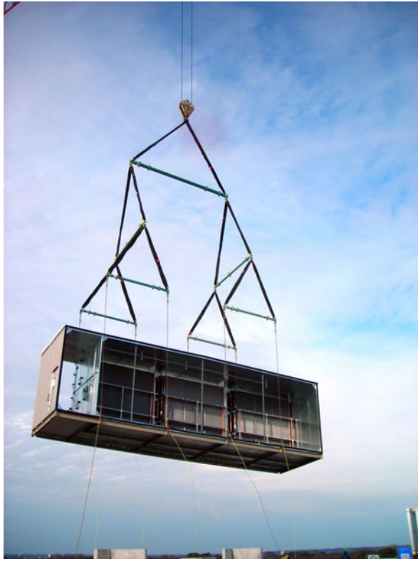
Figure 6. Use proper lifting and rigging methods
