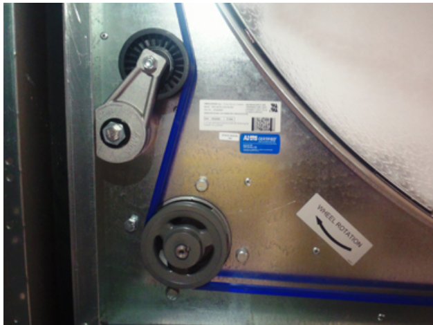
Figure 71. Confirm proper belt tracking on the wheel rim
