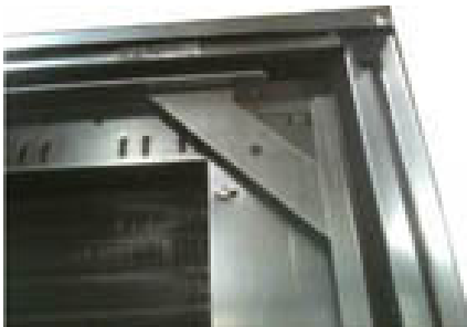
Figure 21. Coil structural gusset
