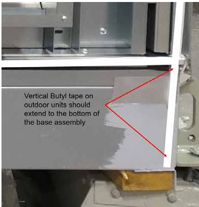
Figure 26. Install outdoor Butyl tape to outermost edge of panel
