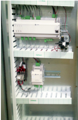
Figure 90. Controller - internally mounted
