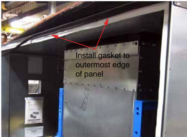
Figure 26. Install outdoor Butyl tape to outermost edge of panel
