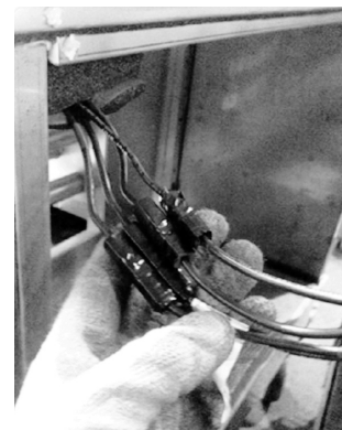
Figure 30. Horizontal section-to-section high voltage quick connects
