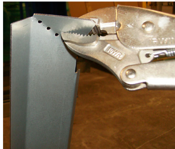
Figure 50. Bend end tabs and apply Butyl tape to flashing
