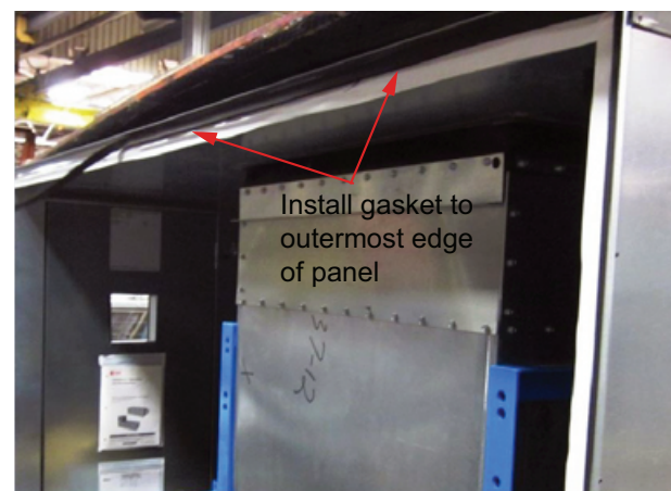
Figure 25. Install gasket to outermost edge of panel
