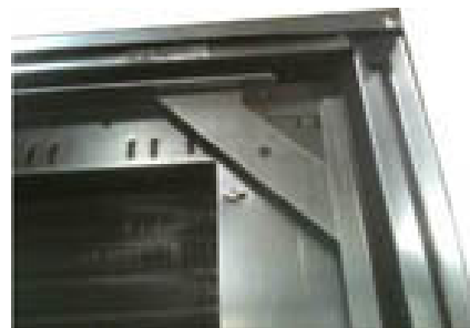
Figure 21. Coil structural gusset
