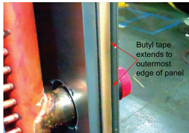
Figure 23. Install gasket to outermost edge of panel
