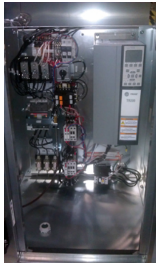
Figure 86. Internally mounted VFD
