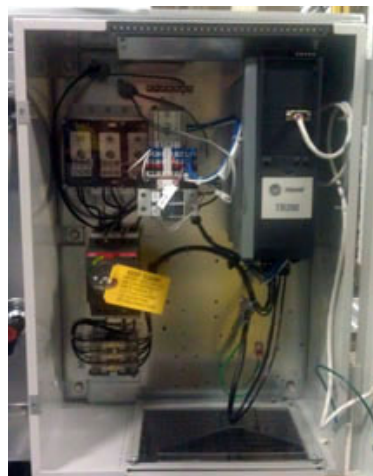
Figure 87. Externally mounted VFD
