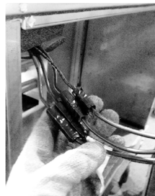
Figure 28. Horizontal section-to-section high voltage quick connects
