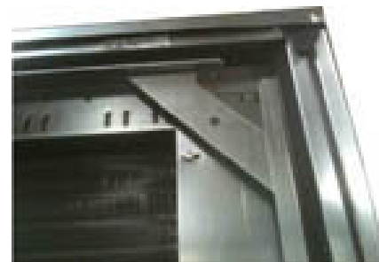
Figure 19. Coil structural gusset
