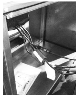
Figure 27. Horizontal section-to-section high voltage quick connects
