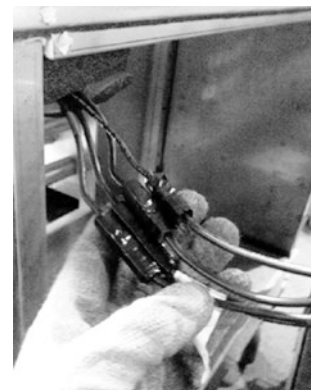
Figure 28. Horizontal section-to-section high voltage quick connects
