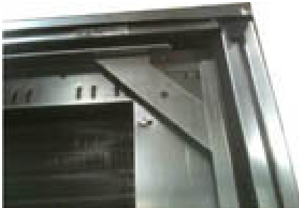
Figure 31. Coil structural gusset
