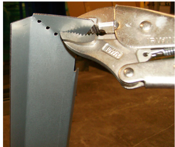
Figure 65. Bend end tabs and apply Butyl tape to flashing
