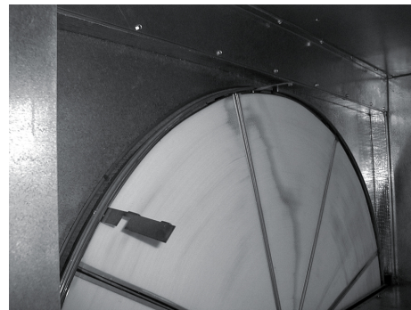
Figure 189. Pull the segment up and out of the wheel frame to remove
