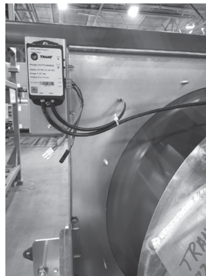
Figure 164. Typical transmitter install for DDP fans
