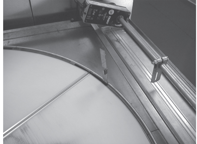
Figure 165. Completely fasten segment retainers
