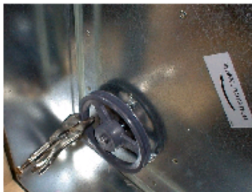
Figure 191. Secure pulley and belt with vise grip to prevent wheel rotation
