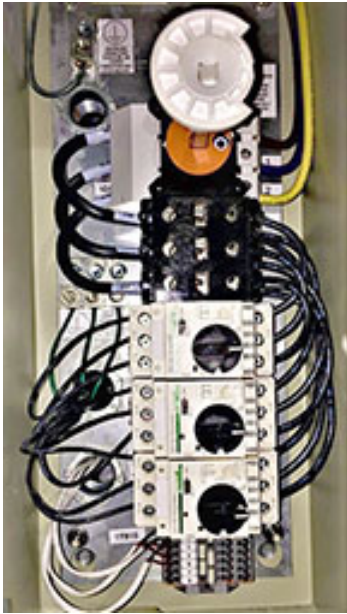
Figure 144. External motorized impeller control panel (MICP)
