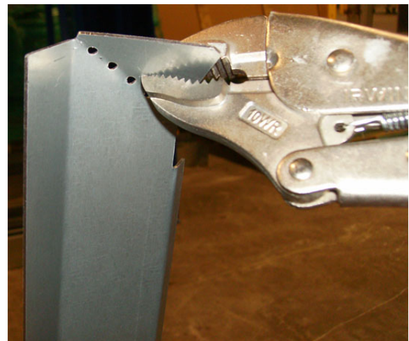
Figure 65. Bend end tabs and apply Butyl tape to flashing
