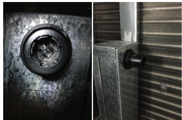
Figure 199. Plug pins into socket, then tighten compression nut
