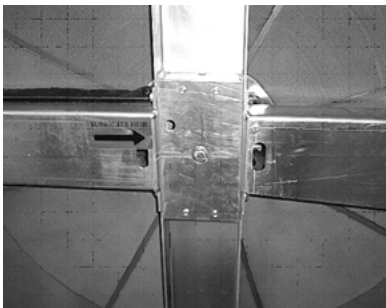
Figure 176. Remove cover plate
