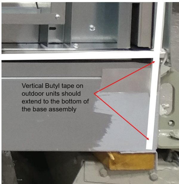
Figure 36. Install butyl tape on outdoor bases
