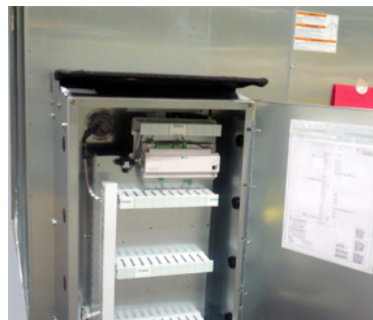
Figure 147. Externally mounted control box
