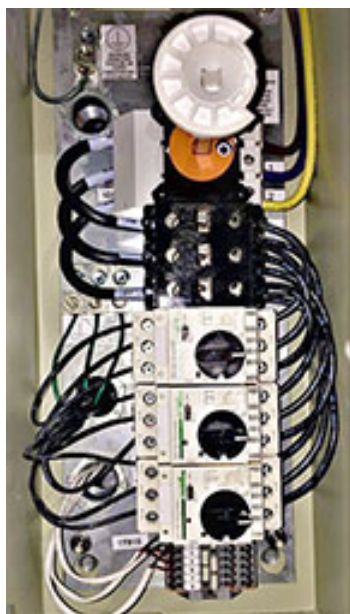
Figure 144. External motorized impeller control panel (MICP)
