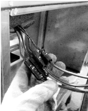
Figure 38. Horizontal section-to-section high voltage quick connects
