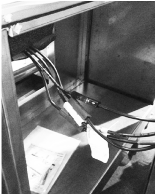
Figure 37. Horizontal section-to-section high voltage quick connects
