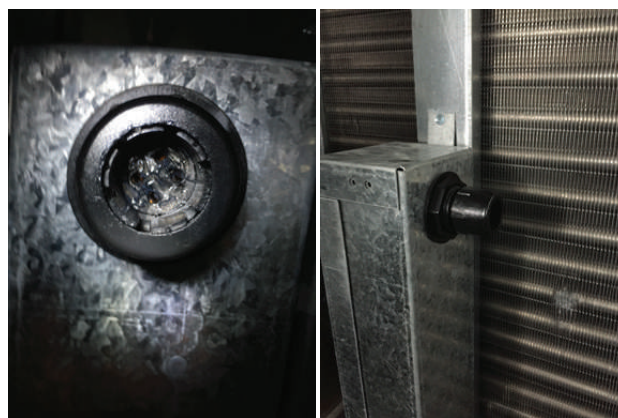
Figure 197. Plug pins into socket, then tighten compression nut
