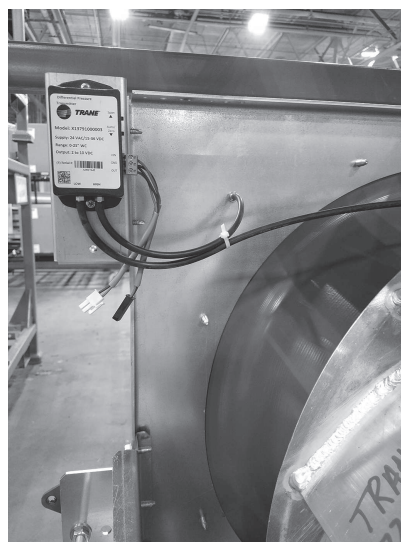
Figure 162. Typical transmitter install for DDP fans
