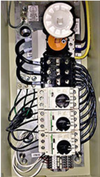
Figure 142. External motorized impeller control panel (MICP)
