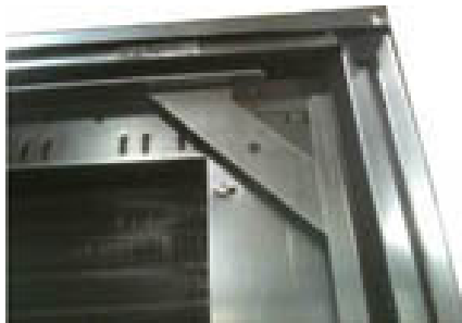
Figure 29. Coil structural gusset
