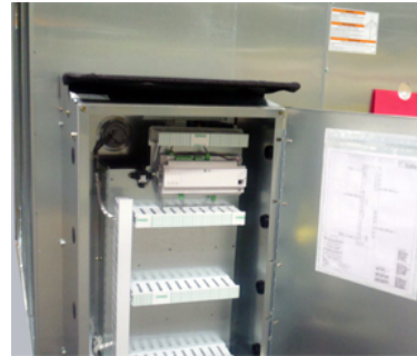
Figure 145. Externally mounted control box
