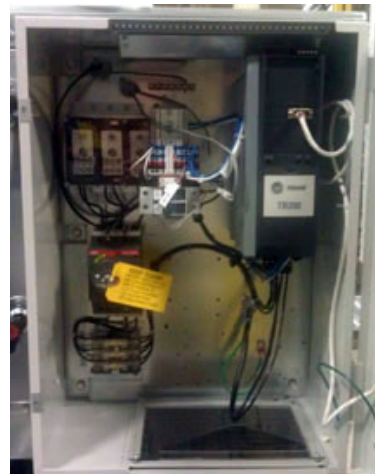
Figure 141. Externally mounted VFD
