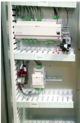
Figure 143. Controller - internally mounted
