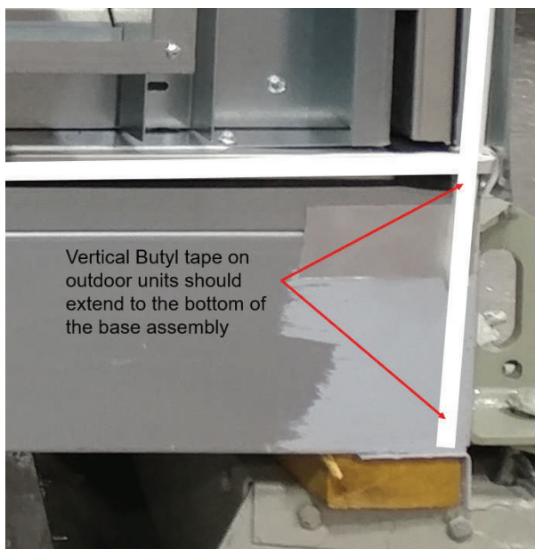
Figure 34. Install butyl tape on outdoor bases
