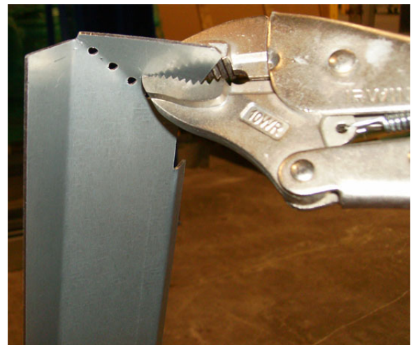
Figure 63. Bend end tabs and apply Butyl tape to flashing
