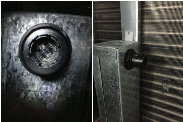
Figure 195. Plug pins into socket, then tighten compression nut
