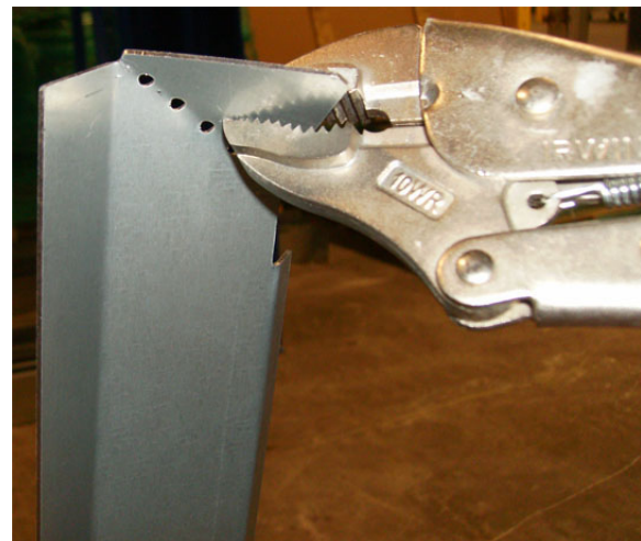
Figure 63. Bend end tabs and apply Butyl tape to flashing
