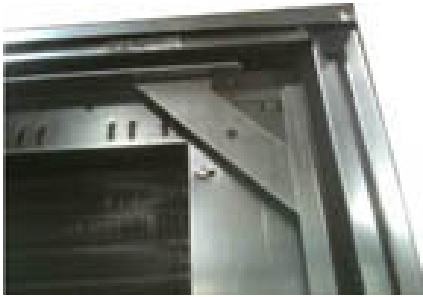
Figure 29. Coil structural gusset
