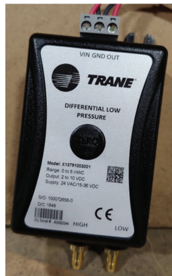
Figure 162. Typical transmitter install for DDP fans
