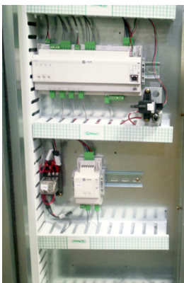
Figure 143. Controller - internally mounted
