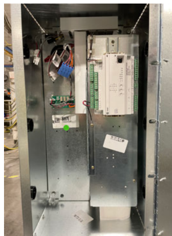
Figure 16. Controller - externally mounted
