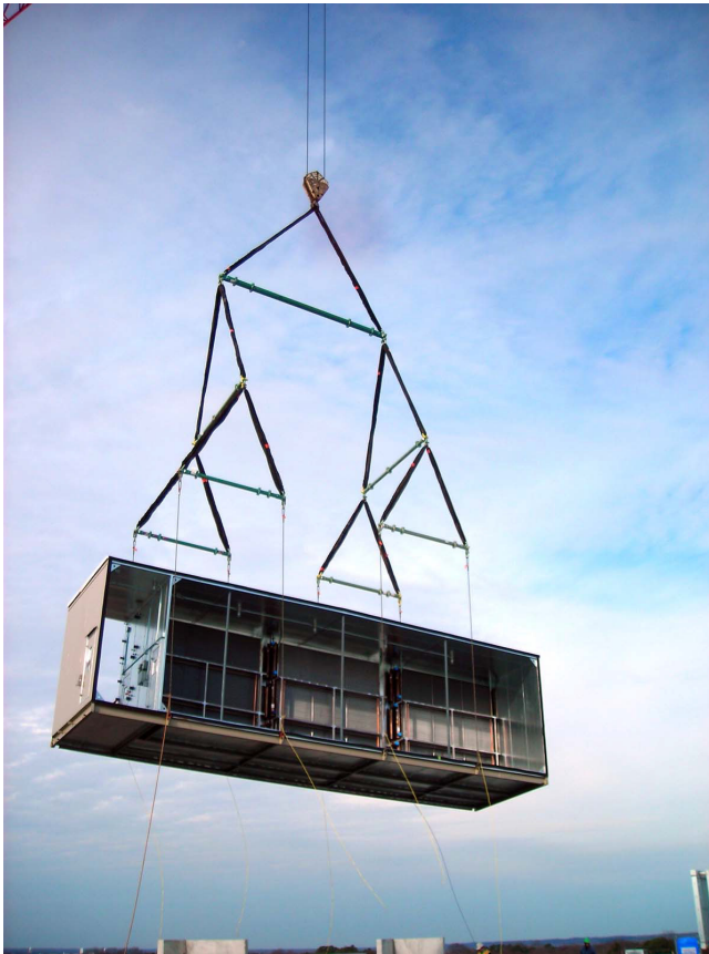
Figure 4. Use proper lifting and rigging methods
