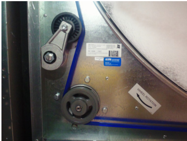
Figure 69. Confirm proper belt tracking on the wheel rim
