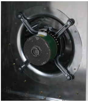
Figure 84. Blower Coil with Trane ECM motor
