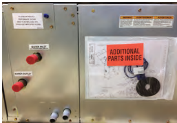
Figure 48. Grommets in accessory bag
