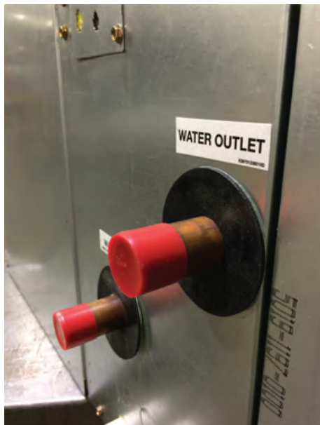
Figure 49. Clean panel before installing grommets
