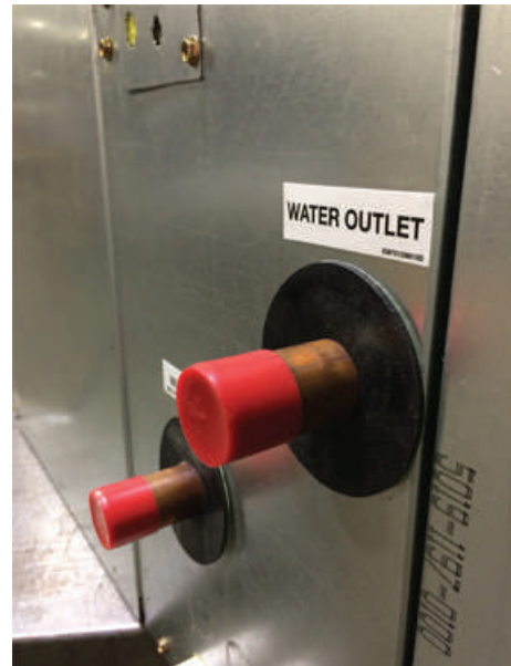
Figure 47. Clean panel before installing grommets
