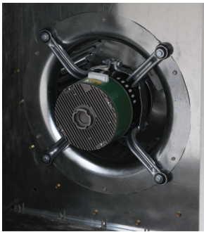
Figure 82. Blower Coil with Trane ECM motor
