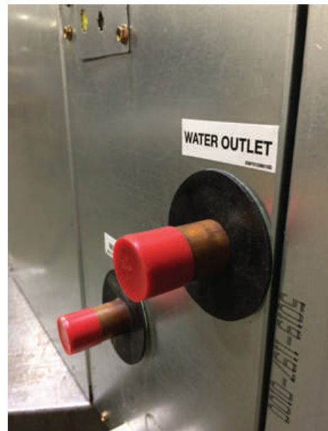
Figure 45. Clean panel before installing grommets
