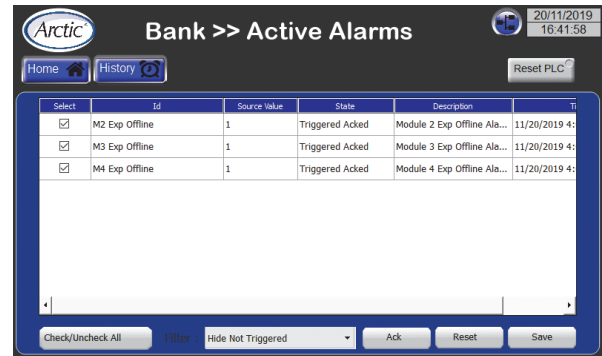
Figure 16. Active alarms for the chiller
