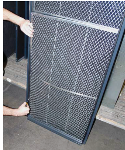
Figure 26. Cleanable filters
