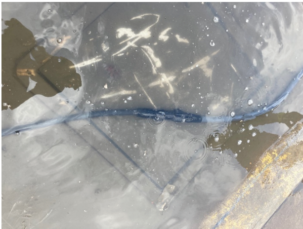
Figure 9. Incorrect installation - submerged cable
