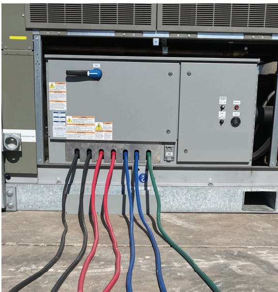
Figure 7. Correct installation - properly spaced cable
