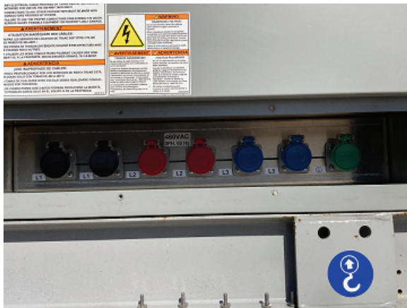
Figure 6. Cam-type connectors without cables connected
