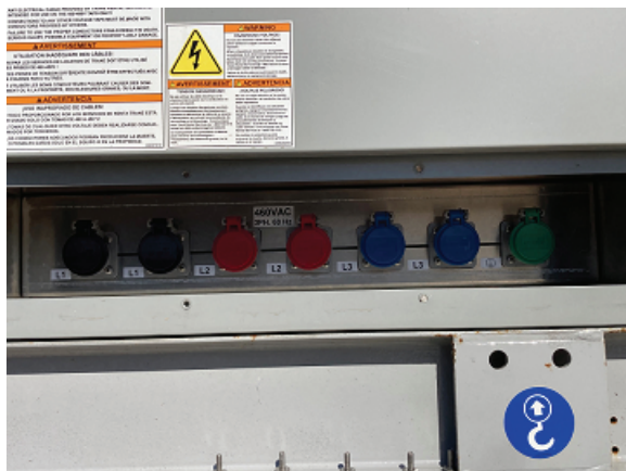
Figure 6. Cam-type connectors without cables connected
