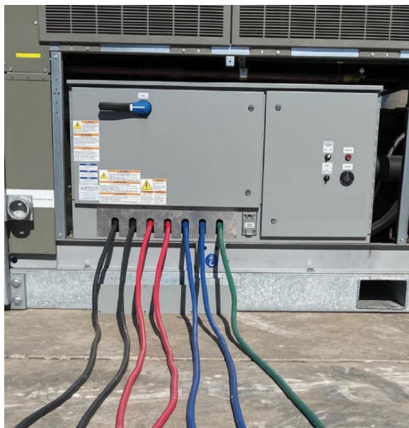
Figure 7. Correct installation - properly spaced cable
