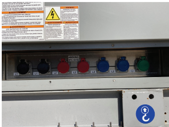
Figure 6. Cam-type connectors without cables connected
